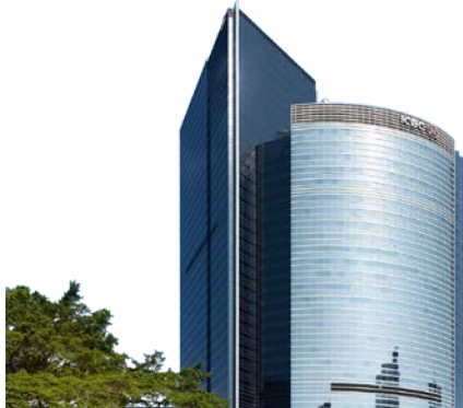
Grade A office complex with GFA 1.6 million sq. ft.
